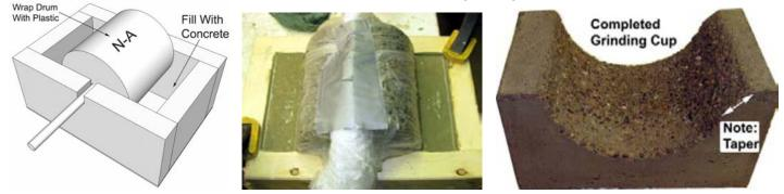
Remove the four sides of the mold when you are comfortable that the concrete is firm but soft enough to scrub to expose the aggregate. Make certain that you scrub from both sides toward the center so as not to damage the edges.
